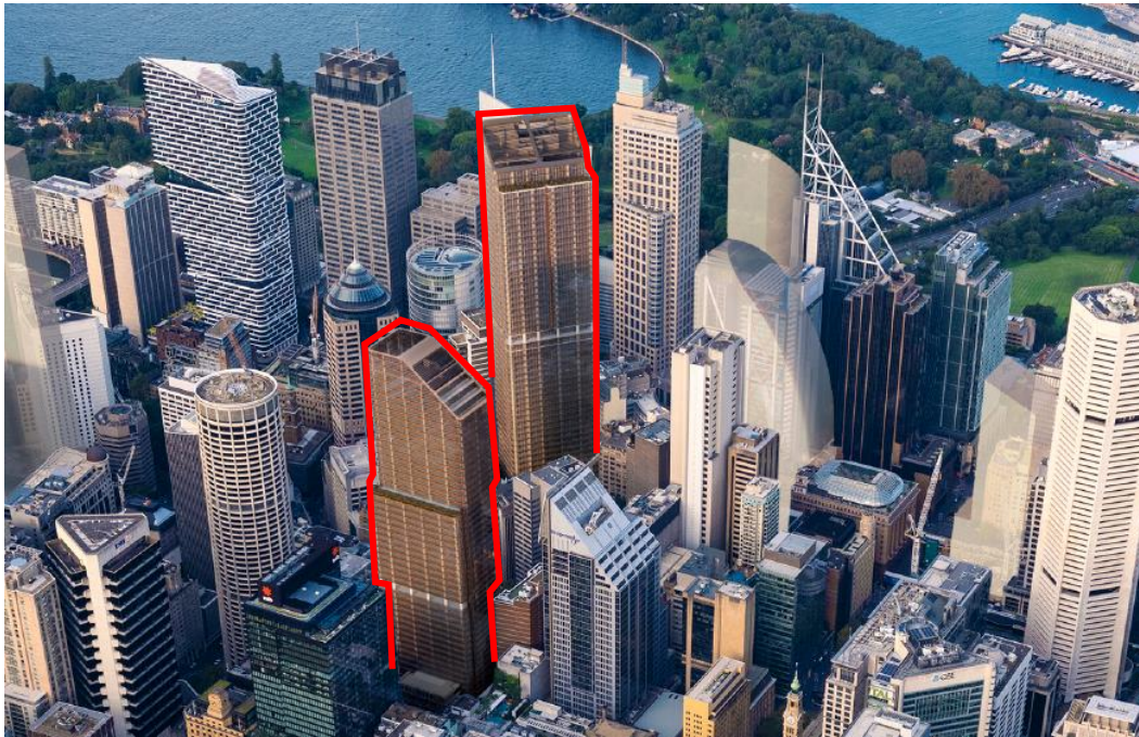
Figure 3: Proponent's reference scheme of the two over-station development towers, outlined in red
